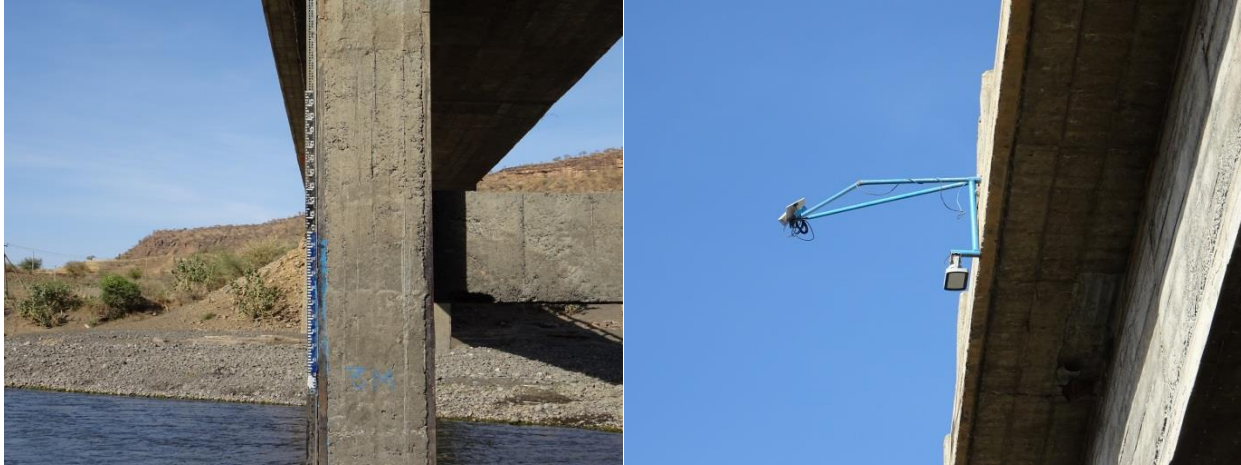
Figure 6: Sensor installed at the bridge of River Zamra for monitoring of depth of the flow (stage).
