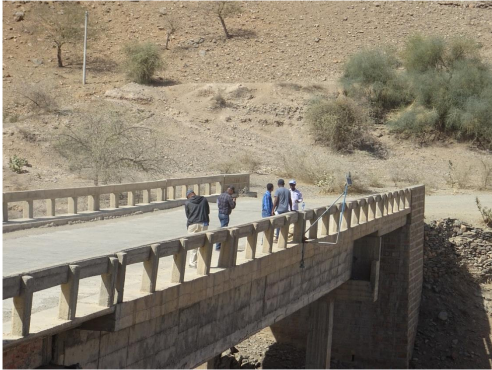
Figure 5: Sensor installed at the bridge of River Zamra for monitoring of depth of the flow (stage).
